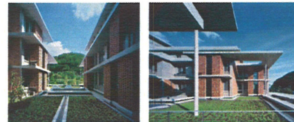
Long eaves and roof planting
