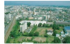
The project site before construction
