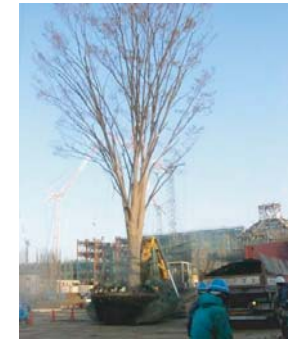
Transportation work of an existing tree
