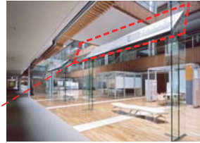
Secondary reflection mirror in A wing atrium
