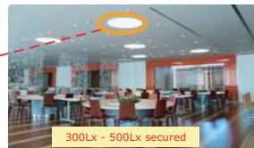
300Lx - 500Lx secured light emitting part of light duct in dining hall
