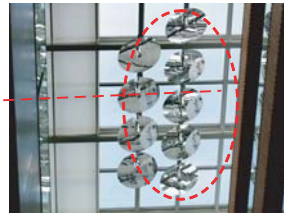
natural sunlight tracking device under A wing atrium top
