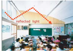
Ordinary Classrooms have Large Windows. Light Shelf guides light to the Interior.
