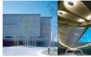
the external wall and ceiling made of pre-cast concrete slabs to reduce the use of form work.
