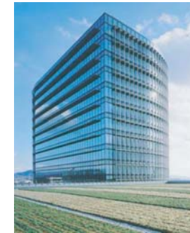
Roof Planting on the Toyota-Hall
